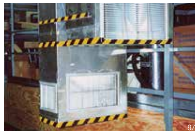
To highlight low hanging objects, protruding equipment, or steps, 3M™ Vinyl Tape 5702 combines yellow and black for a striped combination that calls for attention.
