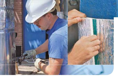
Installing multiple layers of 3M™ Interam™ Endothermic Mat flexible wrap allows you to tailor the desired amount of fire protection — up to 4 hours for structural steel.
