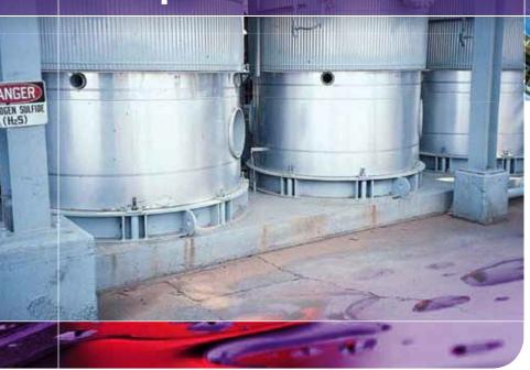
When 3M™ Interam™ Endothermic Mat is applied to vessel skirts and pipe lines, it minimizes the effects of fire exposure by flame impingement in order to reduce the steel's rate of temperature rise and to delay structural failure.
